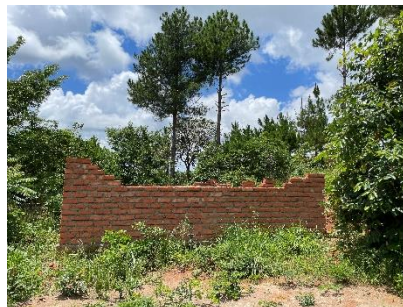
Constructing under five clinic
